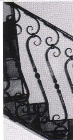
The completed railing with all of the S scrolls the same length, and collars installed. Square head bolts hold the balusters to the railing. The bottom plate is mounted to the rough framing. Rock and plaster will bury the mounting plates.
