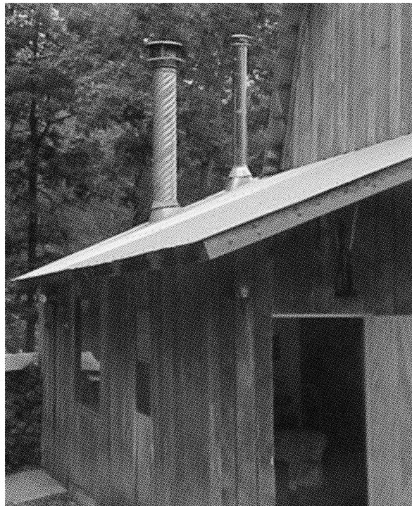
Kent's Shop with his forge stack (15-inch culvert) on left and wood stove stack on right.
